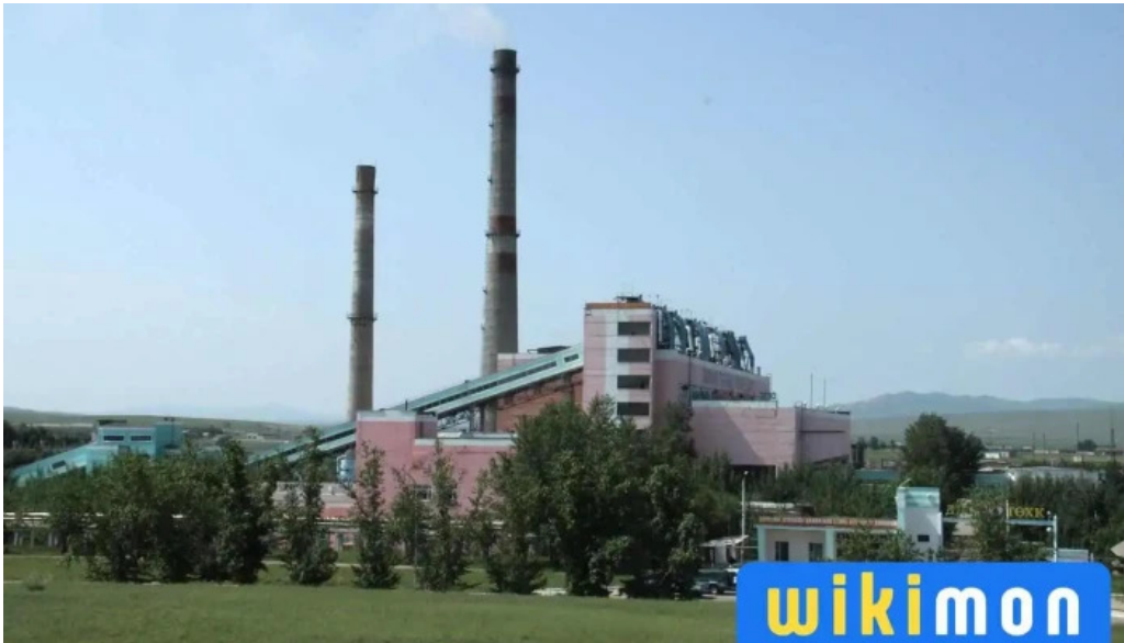
Darkhan thermal power plant ??????
