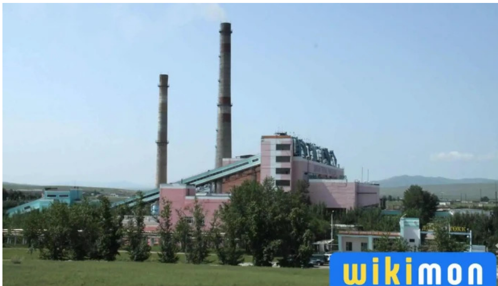
Darkhan thermal power plant bugd
