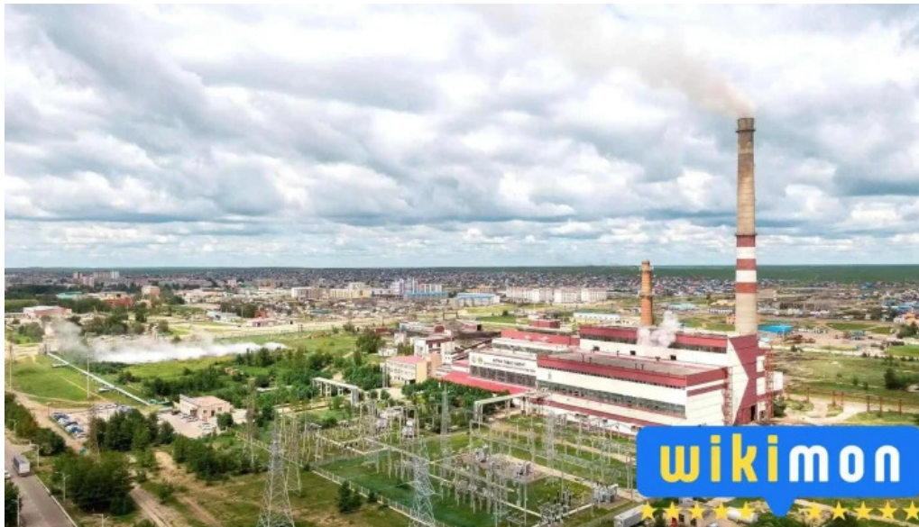
????? eastern energy system ??????????
